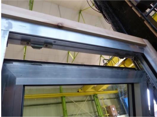
**Figure 5** Scissor stays and keeps on parallel opening sash
