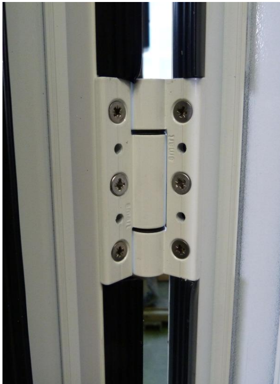
Figure 7 View of non-runner hinge
