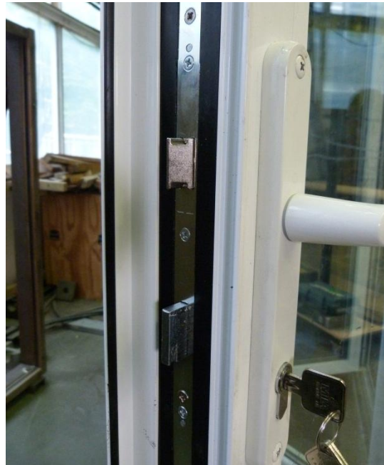
Figure 4 View of deadbolt and latch
