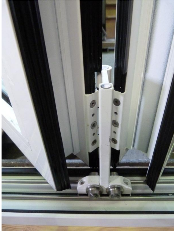
Figure 7 View of non-runner hinge
