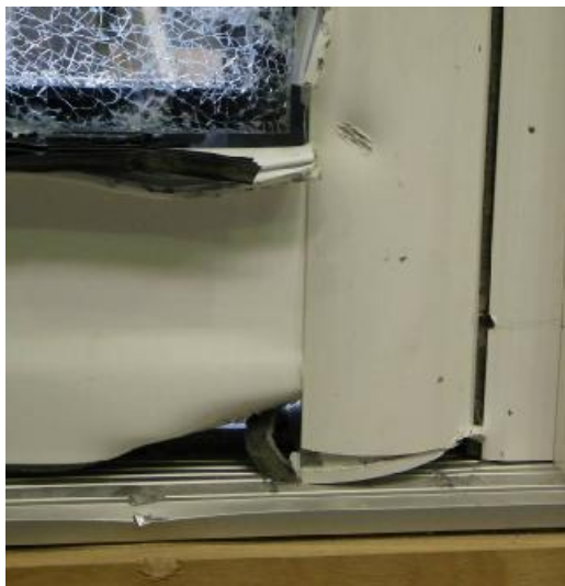
Figure 8 Damage sustained during attack test 7
