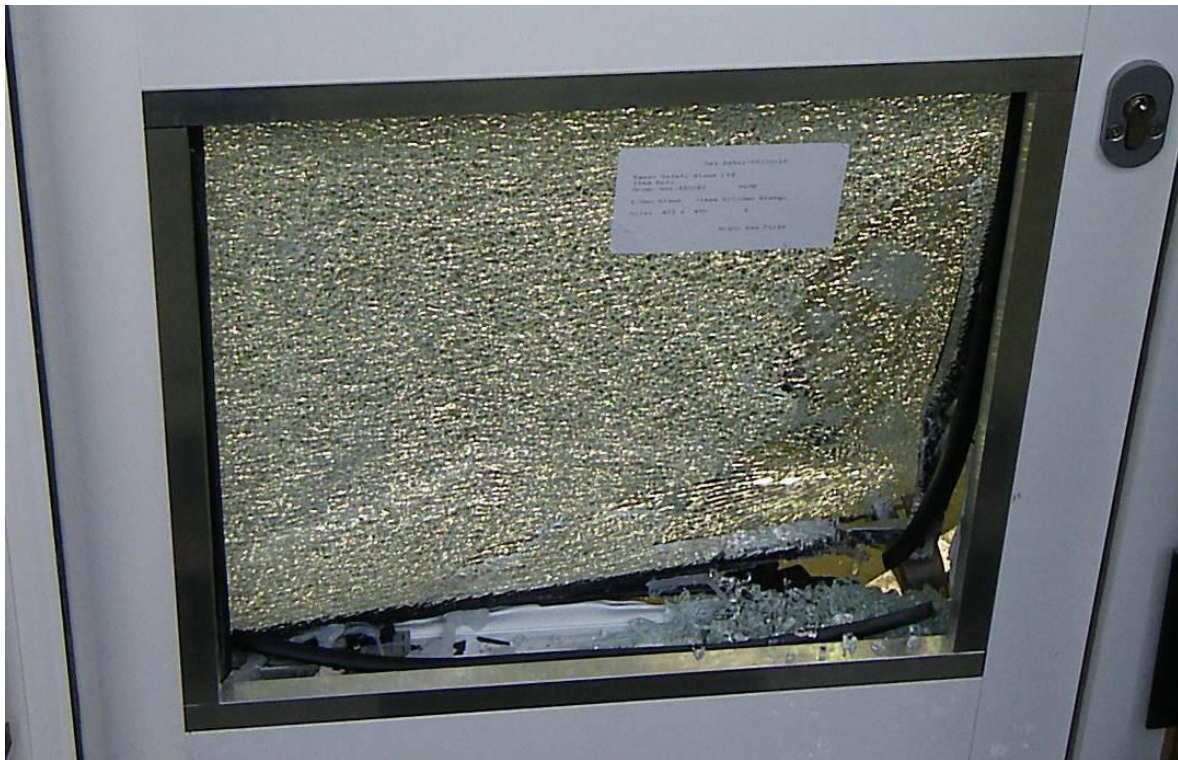
Figure 4 Bottom glazing panel after attack test 2 (lever out glazing panel)
